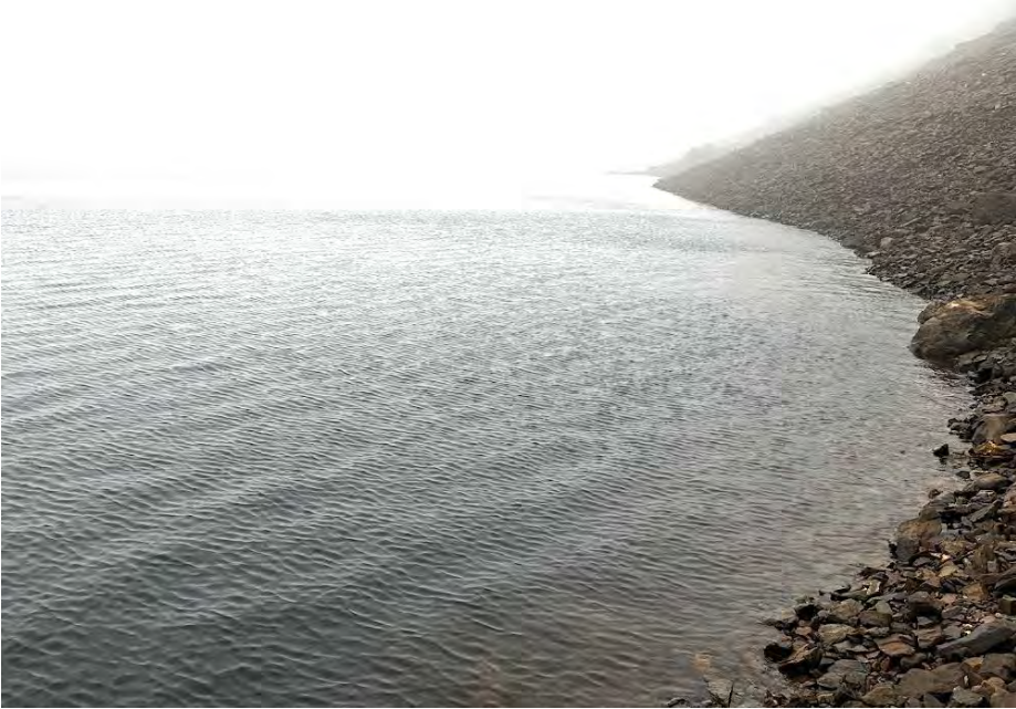
Plate 4: Left bank slope at Loch Sloy
