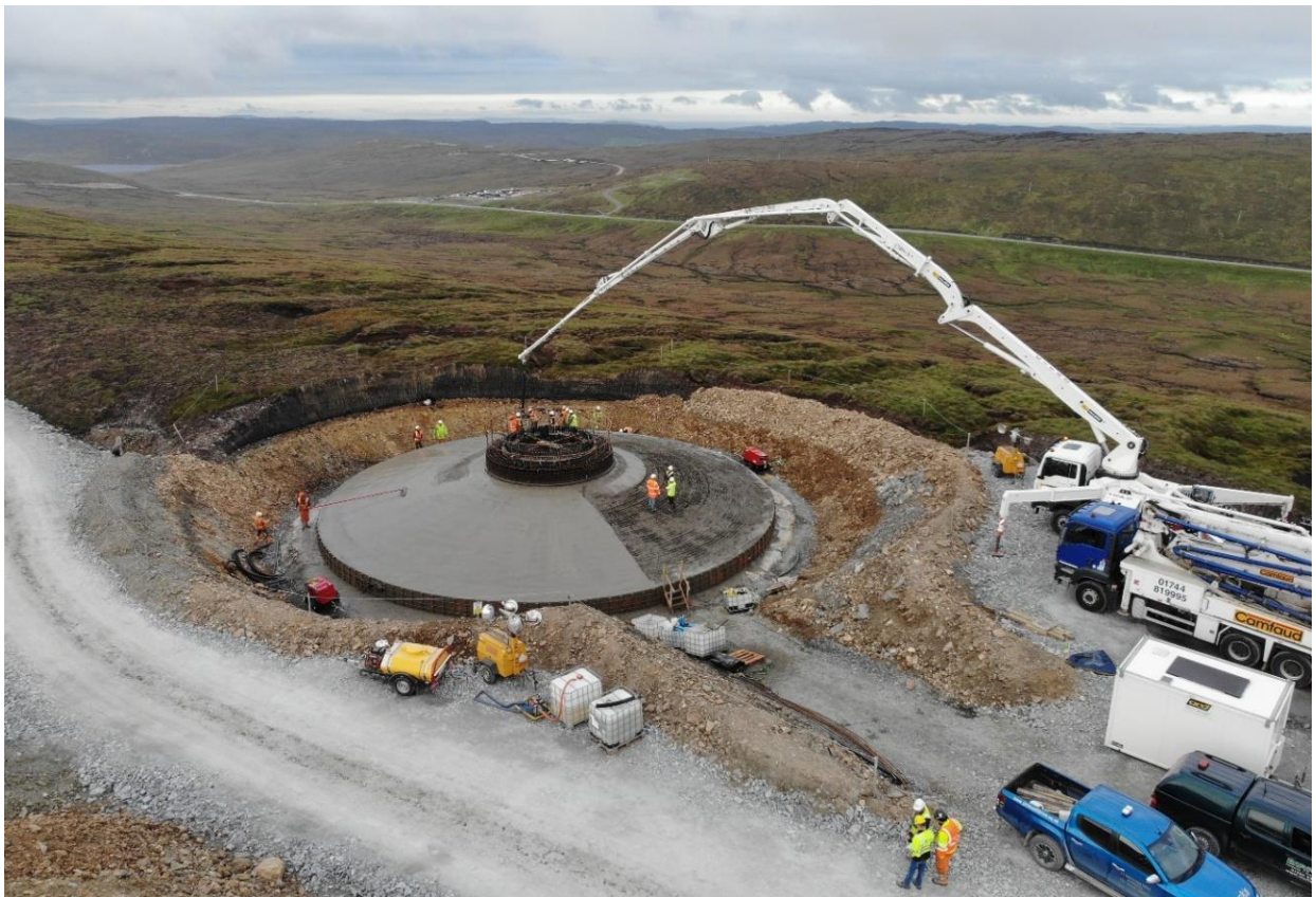
Plate 2-3: WTG Foundation Construction – Concrete Pour
