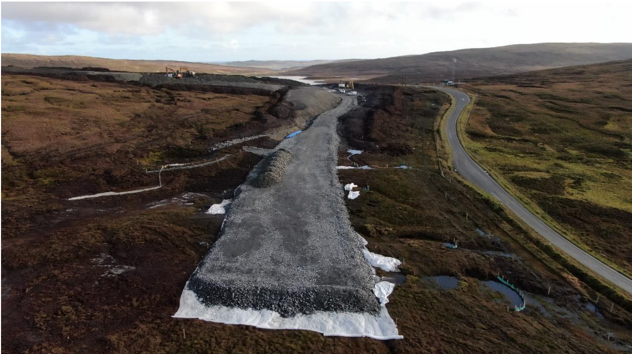
Plate 2-7: Construction of Floating Track
