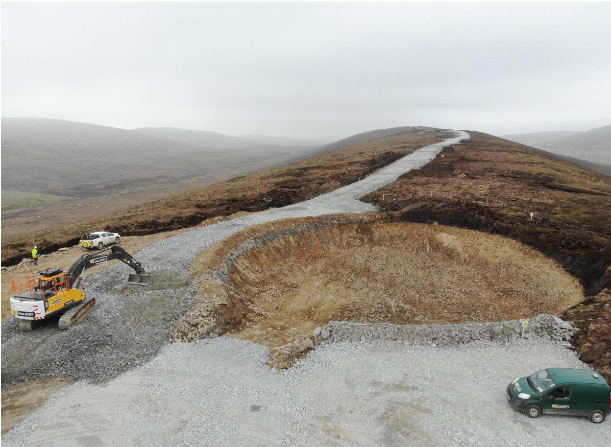
Plate 2-1: WTG Foundation Construction - Excavation
