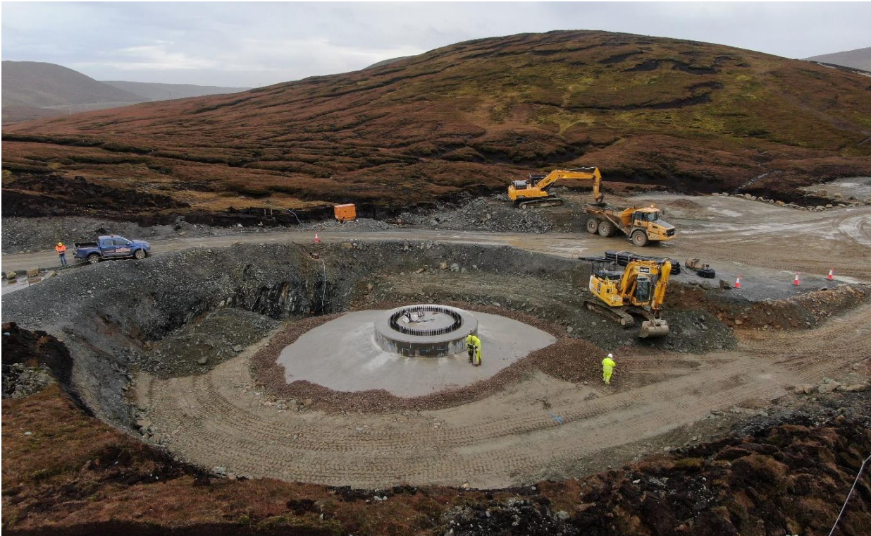
Plate 2-4: Completed WTG Foundation (being backfilled)
