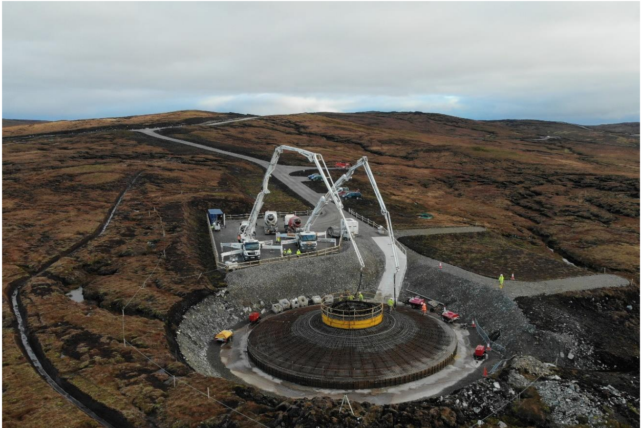
Plate 2-3: WTG Foundation Construction – Concrete Pour
