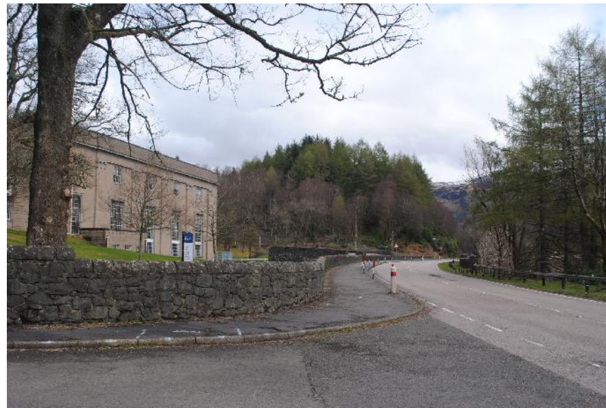
View from A82 looking North
