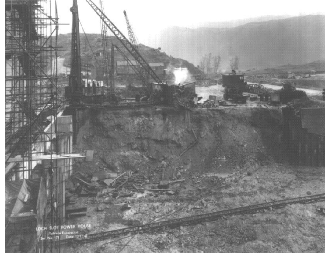
Excavation of Sloy Power Station tailrace during construction. Photograph taken circa 1949.
