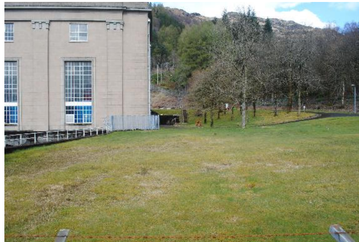
View from A82 of proposed area for pump building
