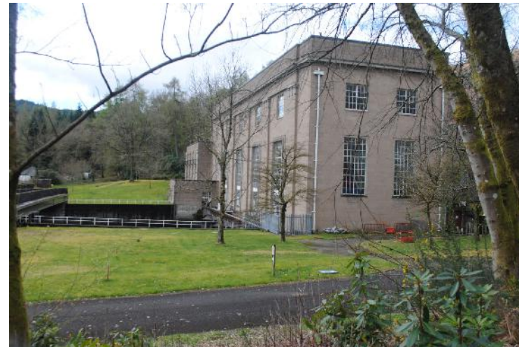
View from woodland to the North of location for proposed pump building.
