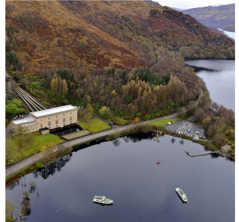
Sloy Hydro Scheme viewed from the south east as existing. Image Credit SSER
