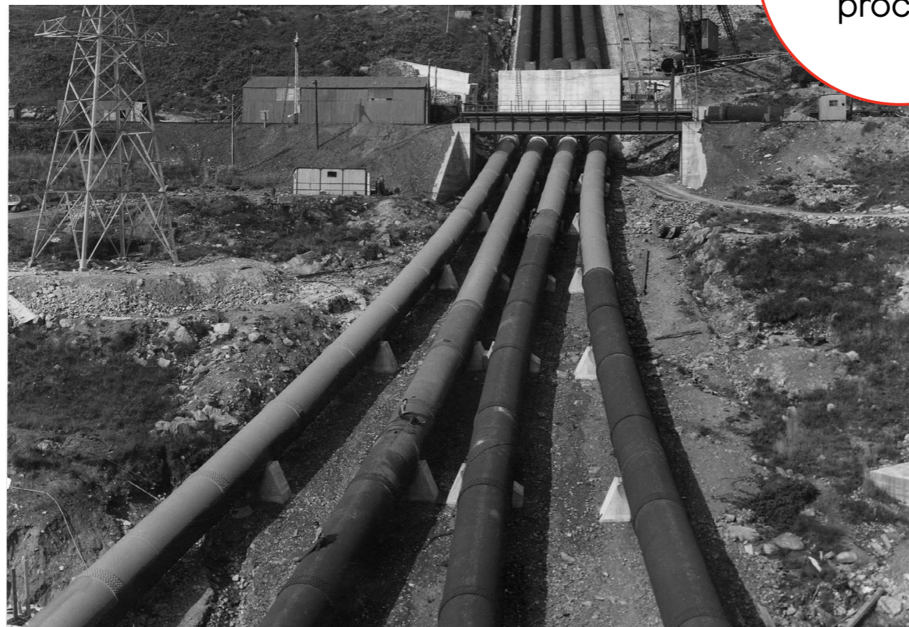
View of the penstocks during construction; Image Credit: SSER
