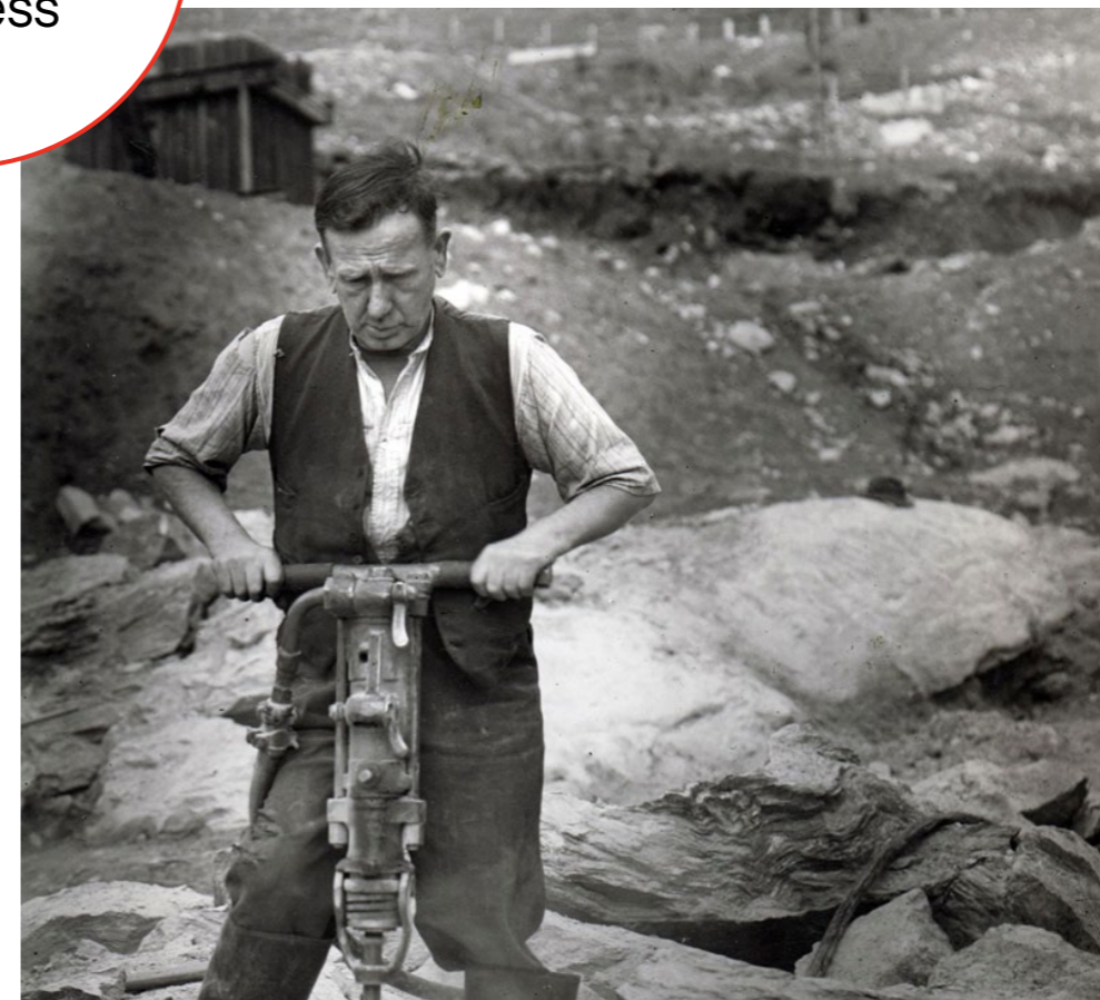
Worker on site during construction; Credit: SSER
