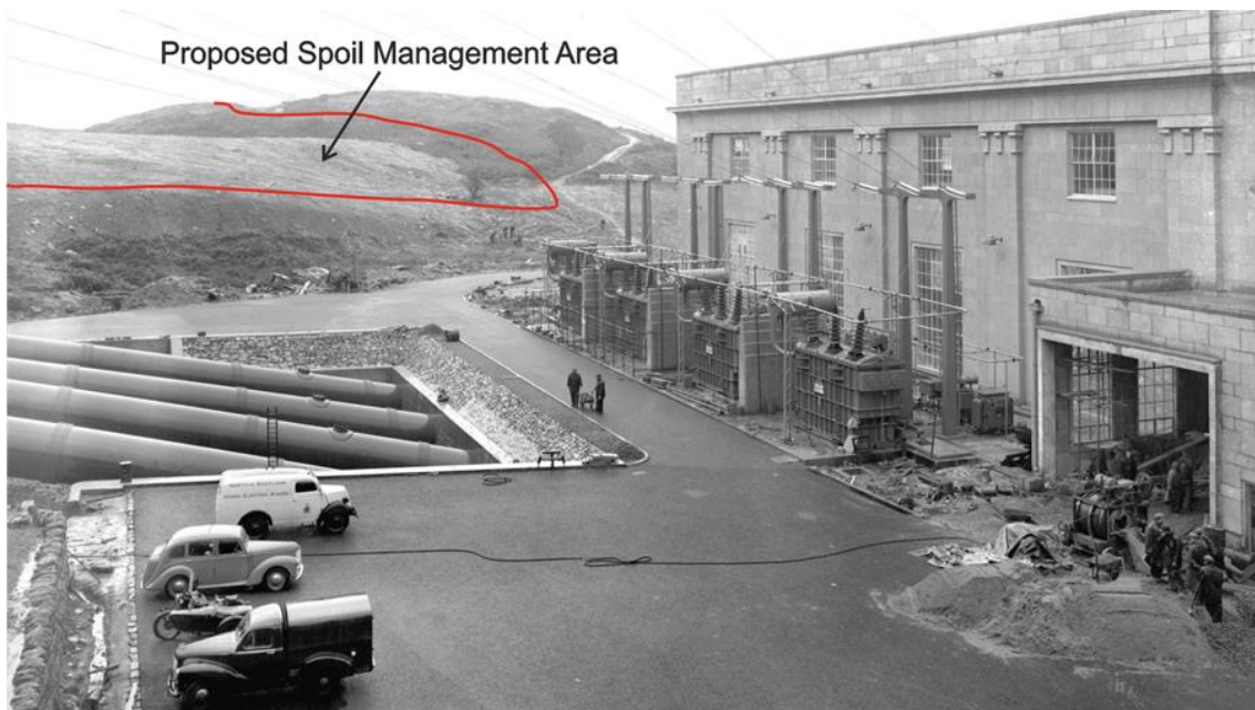
Plate 5: View of the rear of Sloy Hydroelectric Power Station during construction circa 1950 (Photo Credit: SSE Renewables).
