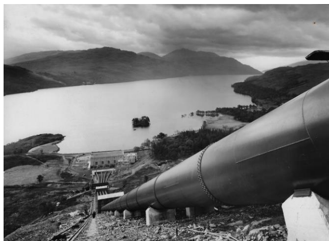
Plate 15.1: View of Sloy Power Station construction works from the west (c.1940)
