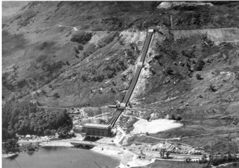
Plate 15.2: View of Sloy Power Station construction works from the east (c.1940)
