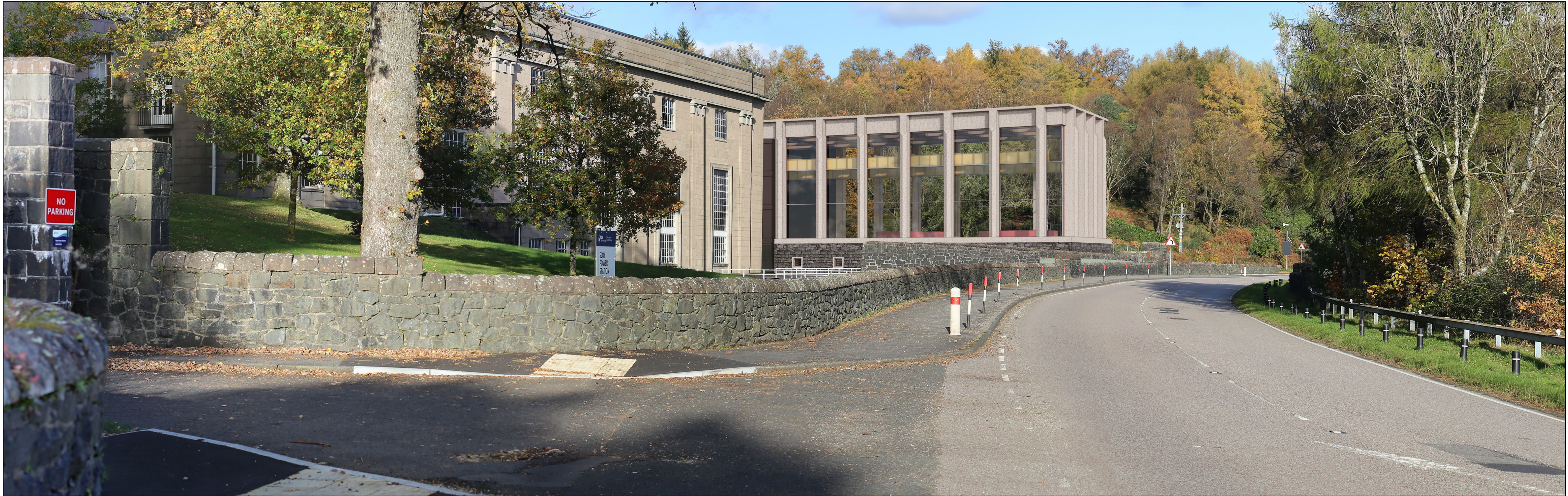
VL2. View from the A82, south of Sloy Hydroelectric Power Station - Photomontage - Fig 4.6c
