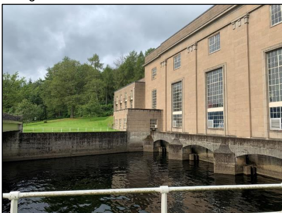
Photo 11: Open standing water and power station building
